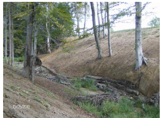
Site after restoration
